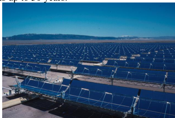
Fig. 1.2. Solar thermal power plant “ Solar Energy Generating Systems ” in California with a capacity of 354 MW
